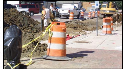
(Photo by Clara Osten) Crews from M.E. Collins work to remove dirt on West First Street before water mains and storm sewers are replaced.
